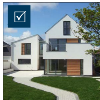
Design Cue - house in Portrush, Northern Ireland. Prominent projecting gable with elements of a lower height set back.
